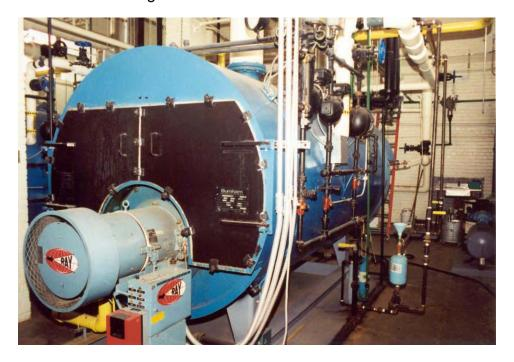
Figure 6-1 Hot Water Boiler
