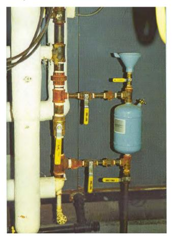
Figure 8-1 Chemical Pot Feeder
