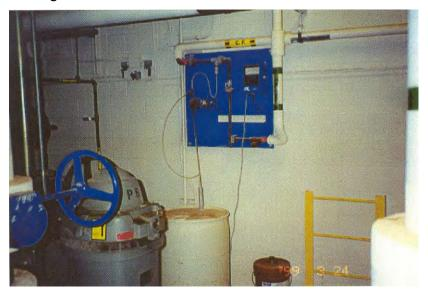
Figure 8-4 Automatic Neat Chemical Feed
