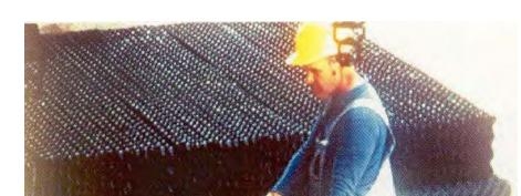
Figure 5-11 High-Efficiency Cooling Tower Film Fill
