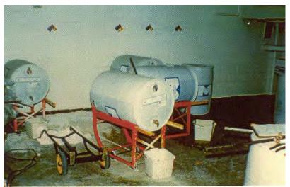
Figure 8-2 Manual Chemical Feed System
