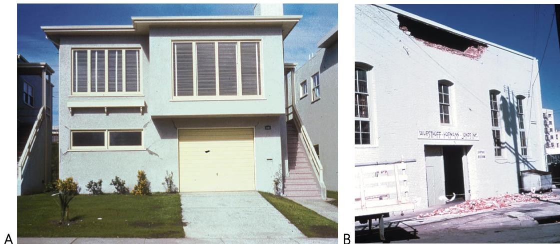
**Figure 2-9.** Many damaged buildings can be safely occupied. (A) A wood-frame dwelling with cracked stucco at door and window corners would probably be evaluated green, “inspected.” (B) An unreinforced masonry warehouse with parapet damage over one of several entrances could nonetheless be used if the entrance beneath the damaged parapet were not used. (Images: public domain)
