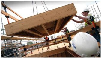
B) LANDING OF A PREFABRICATED FLOOR CASSETTE
