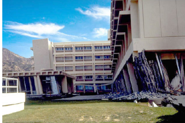
Excessive Drift at the Soft Ground Story of the Olive View Hospital in the 1971 San Fernando EQ (from FEMA P-2156 and William Godden, NISEE-PEER)
