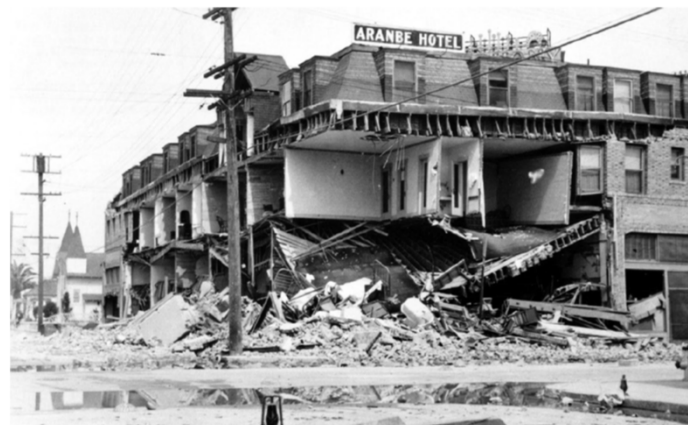
URM Bearing Wall Damage in the 1933 Long Beach EQ (from FEMA P-2156 and Los Angeles County Library)
