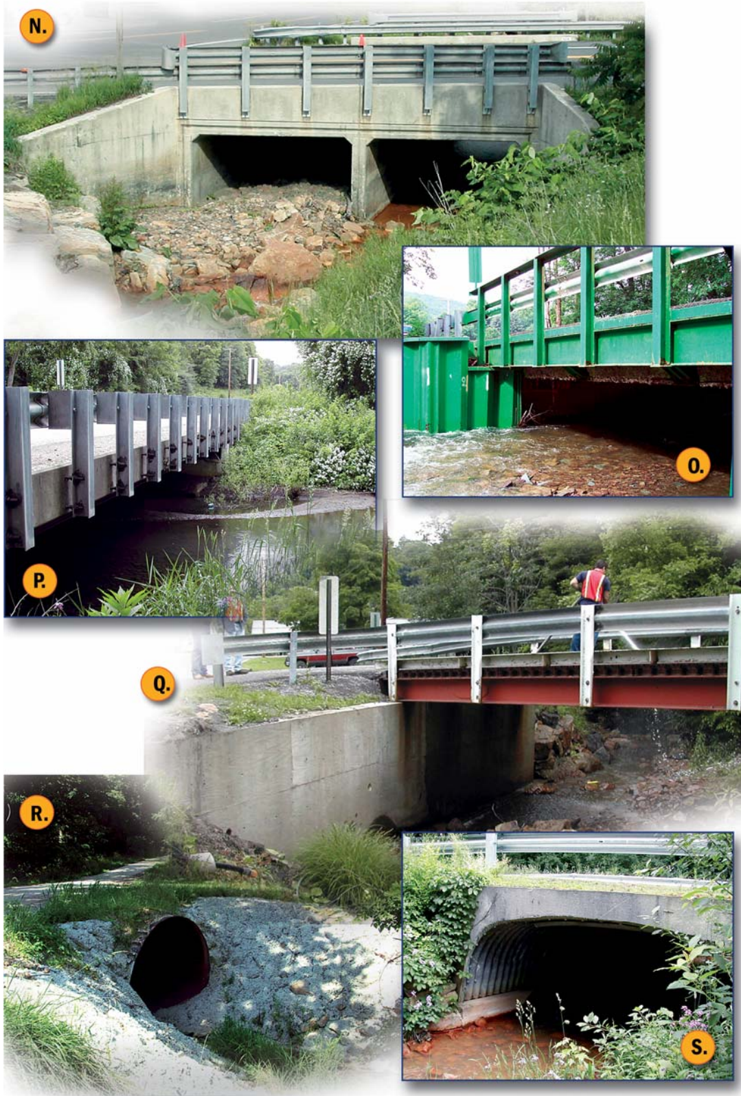
Figure 2-3. Typical Bridges, Culverts and Low-water Crossings
