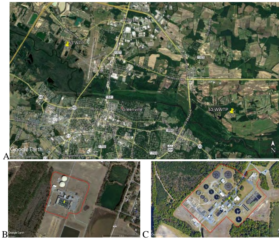
Figure 6-19: A. Water treatment plant (denoted 53 WTP) and wastewater treatment plant (denoted 53 WWTP) sites in Greenville, North Carolina. B. Image of the water treatment plant, with berm highlighted in red. C. Image of the wastewater treatment plant.
