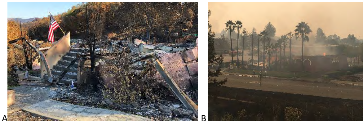
Figure 2-68: (A) Houses and (B) commercial buildings burned in the 2017 Tubbs Fire. (Image credits: (A) Frank Schulenberg 2017, (B) ATS 2017, both CC BY-SA 4.0)
