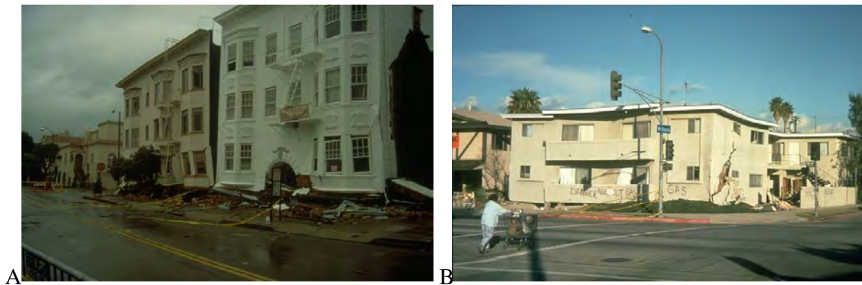
Figure 2-50: Examples of collapsed soft-story wood-frame multifamily dwellings. (A) Collapsed apartment buildings in the San Francisco Marina District after the 1989 Loma Prieta earthquake (Image credit: R.B. Seed, 1989, via UC Berkeley NISEE, with permission). (B) Apartment building collapse after 1994 Northridge earthquake, associated with soft-story conditions (Image credit: UC Berkeley NISEE, 1994, with permission).
