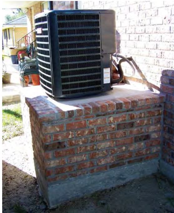
Figure 2-41: An example of an elevated air conditioning unit. (Source FEMA P-348 – Figure 3-1)
