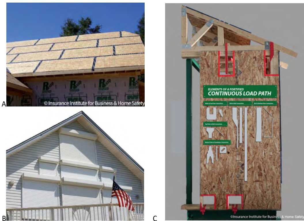
Figure 3-2: Examples of retrofit measures required by IBHS (A) Sealed roof deck over seams between roof sheathing, as required for FORTIFIED Roof. (B) Shutter installation required for FORTIFIED Silver. (C) Continuous load path required for FORTIFIED Gold. (photos used with permission from IBHS)
