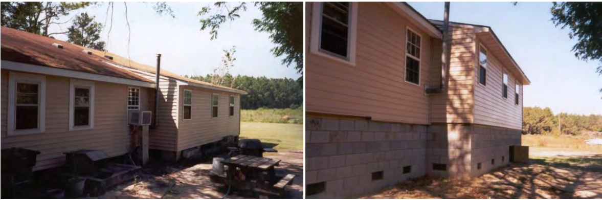
Figure 2-33: Before (left) and after (right) elevation photos for a single-family house (Source: Stacy Wright)
