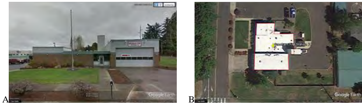
Figure 5-18: Gresham Fire Station 74 (A) in Google Earth Street View, and (B) from above.
