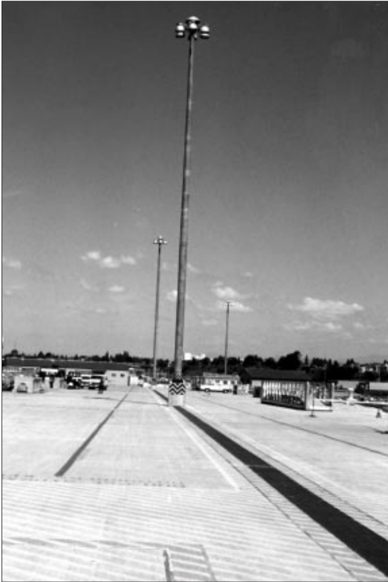
For ease of maintenance, these highly efficient lights can also be lowered to the ground.
