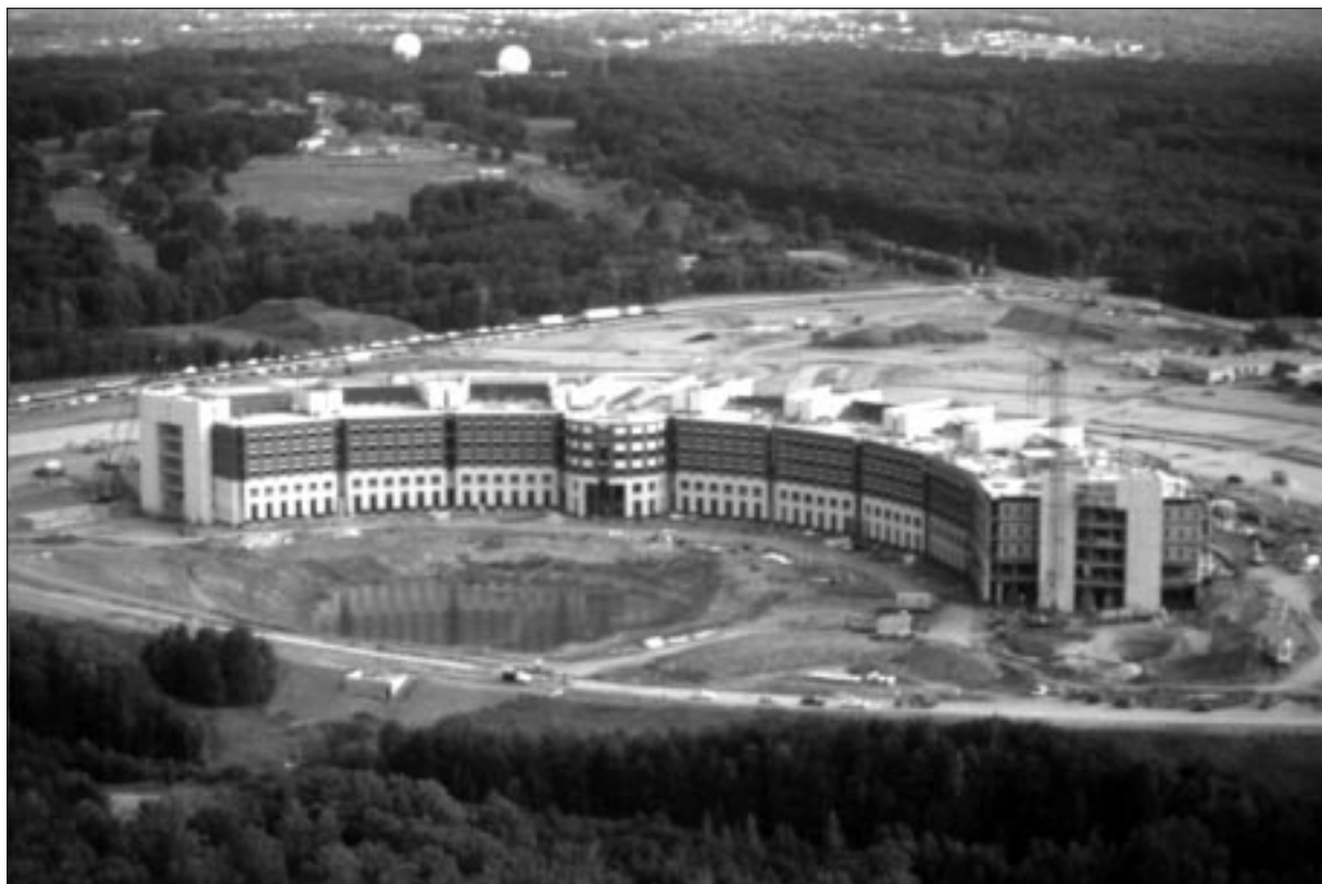
Early CAD layouts indicated that there was insufficient space in the original design. Two modules were added.
