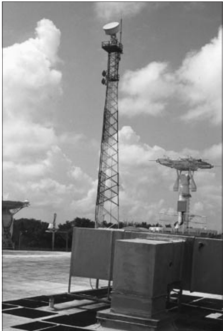
Redundancy is mission essential; maintenance of the MILA antennas is one of the most important jobs.
