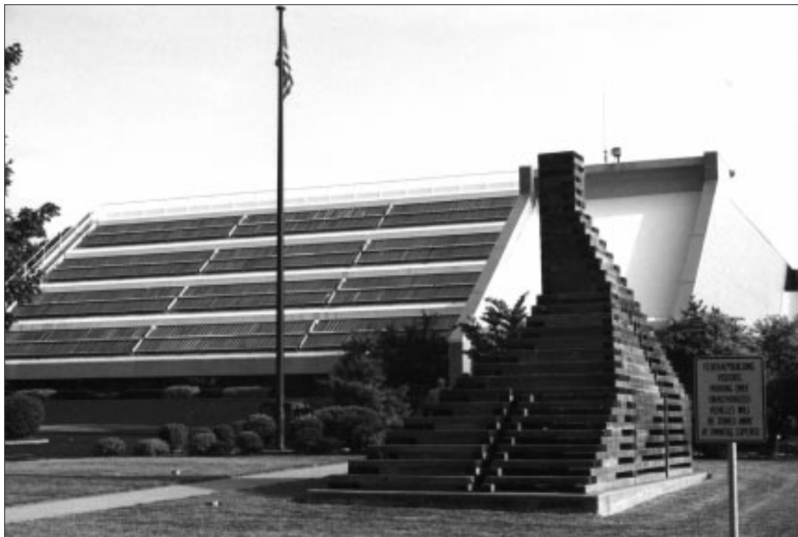
Wooden sculpture at entry was not sufficient to protect the vulnerable solar arrays.
