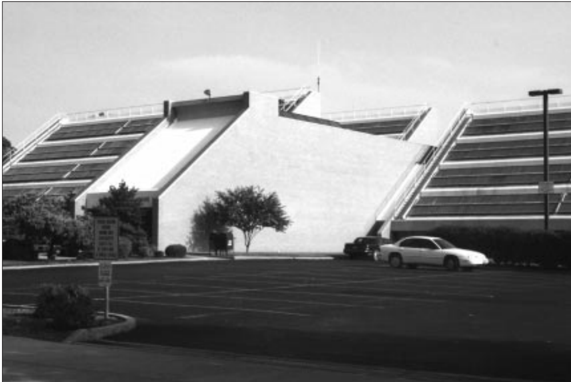
Solar arrays dictated the design of the south elevation of the Federal Office Building in Carbondale, Illinois
