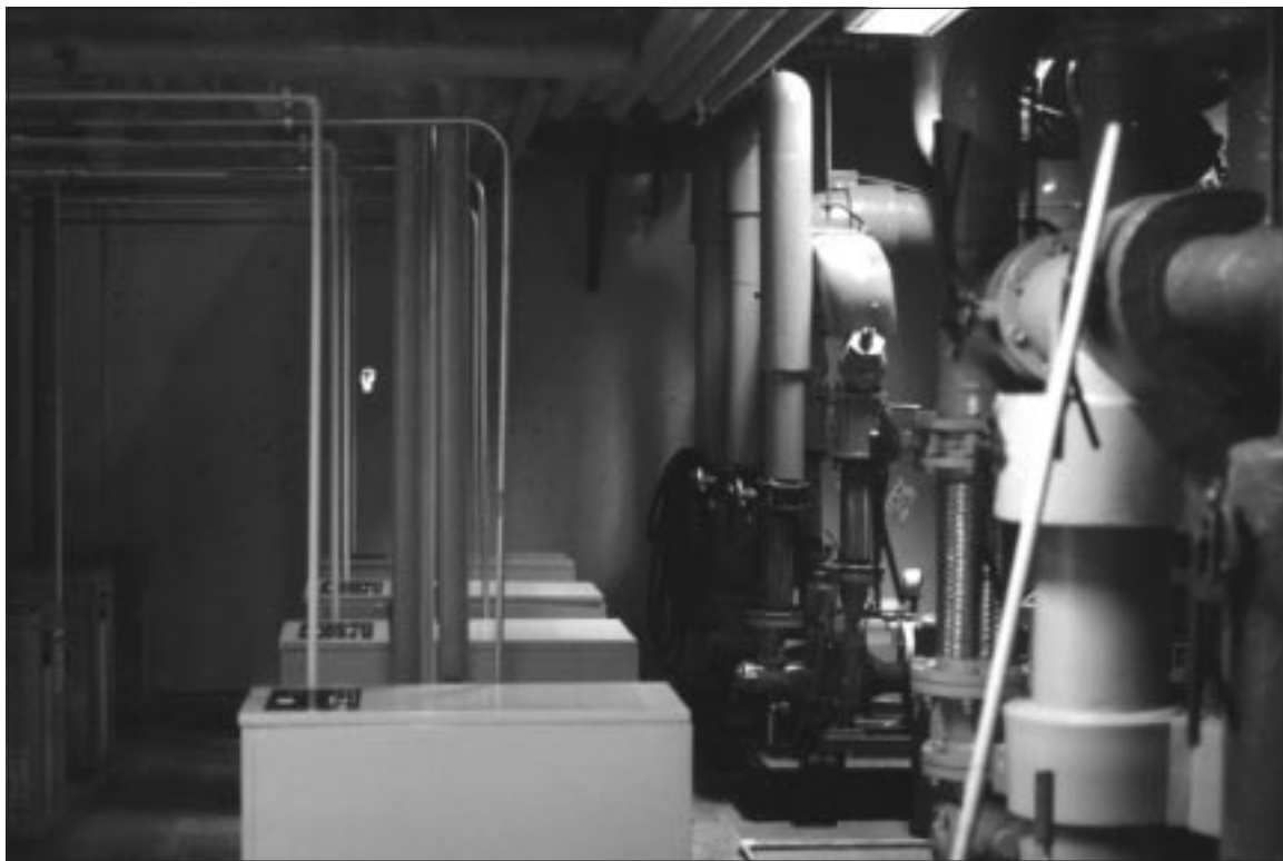
New packaged boilers are able to satisfy varying demand much more efficiently.
