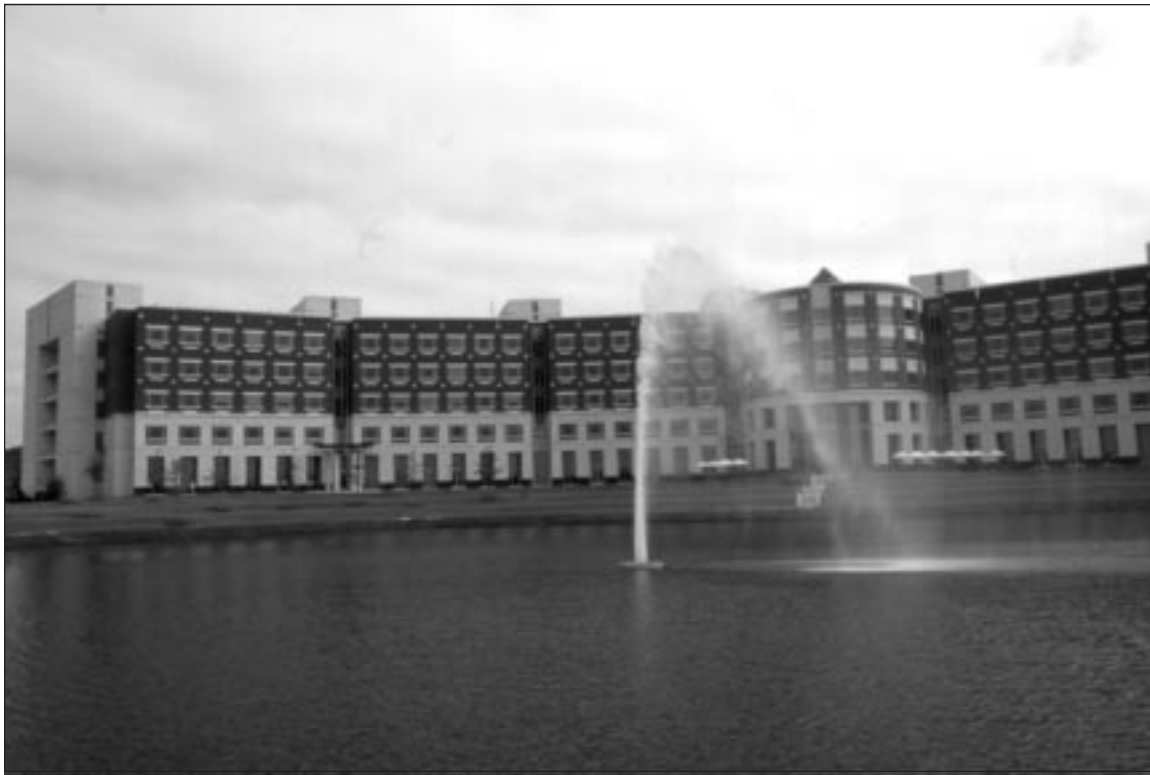
Aeration of the retention pond, which collects parking lot runoff, allows it to be used to water landscaping.
