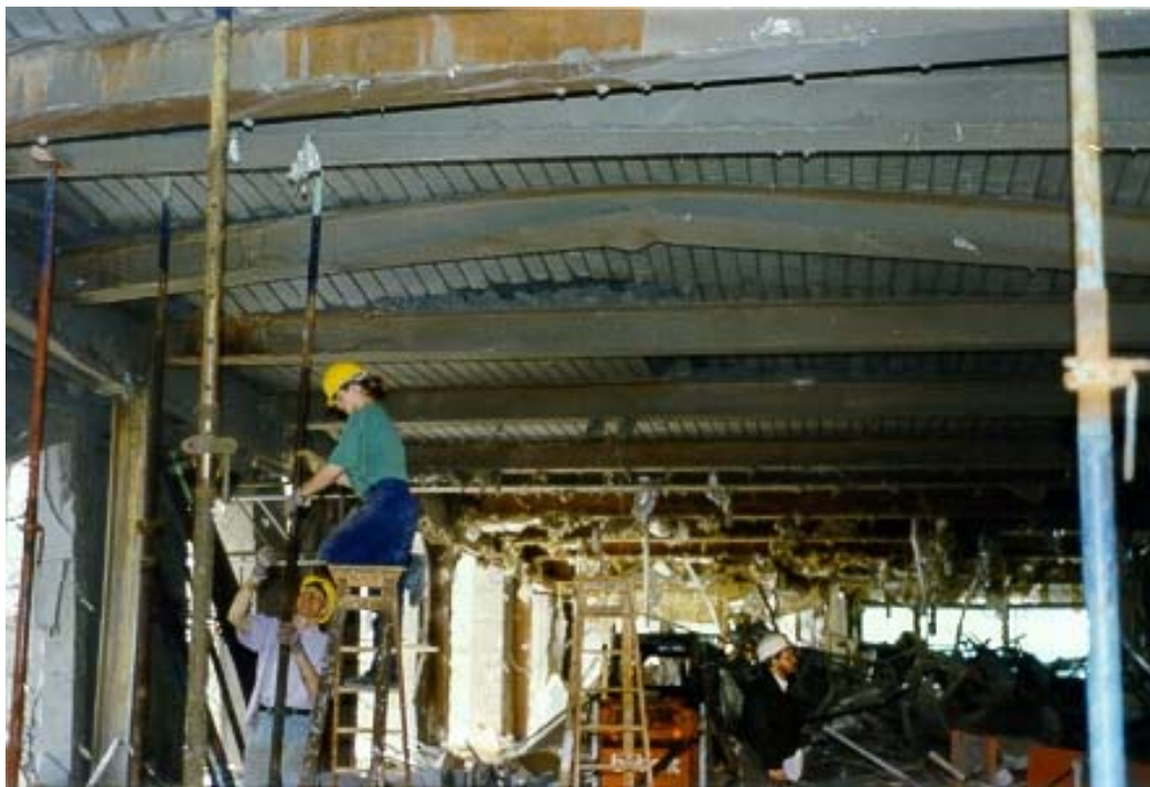
Figure 2. Damage to ground floor steel columns – Exchequer Court, St. Mary's Axe
