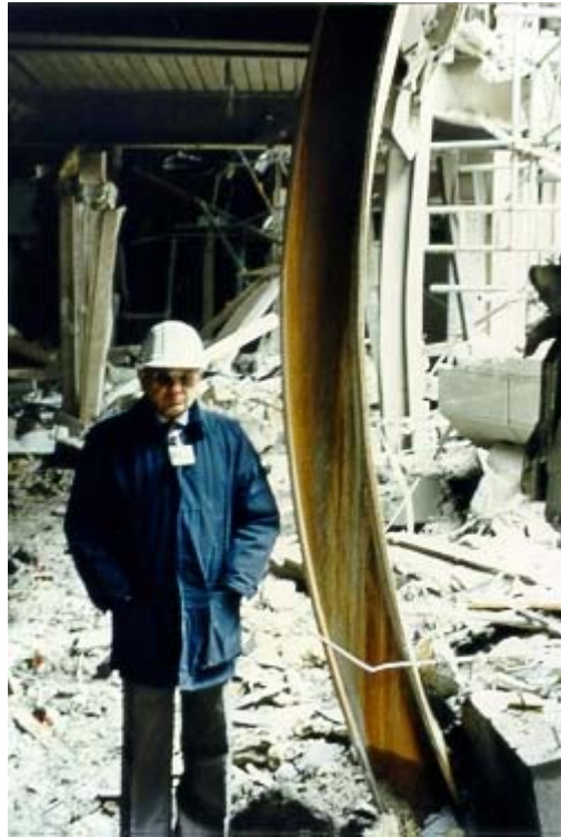
Figure 2. Damage to ground floor steel columns – Exchequer Court, St. Mary's Axe
