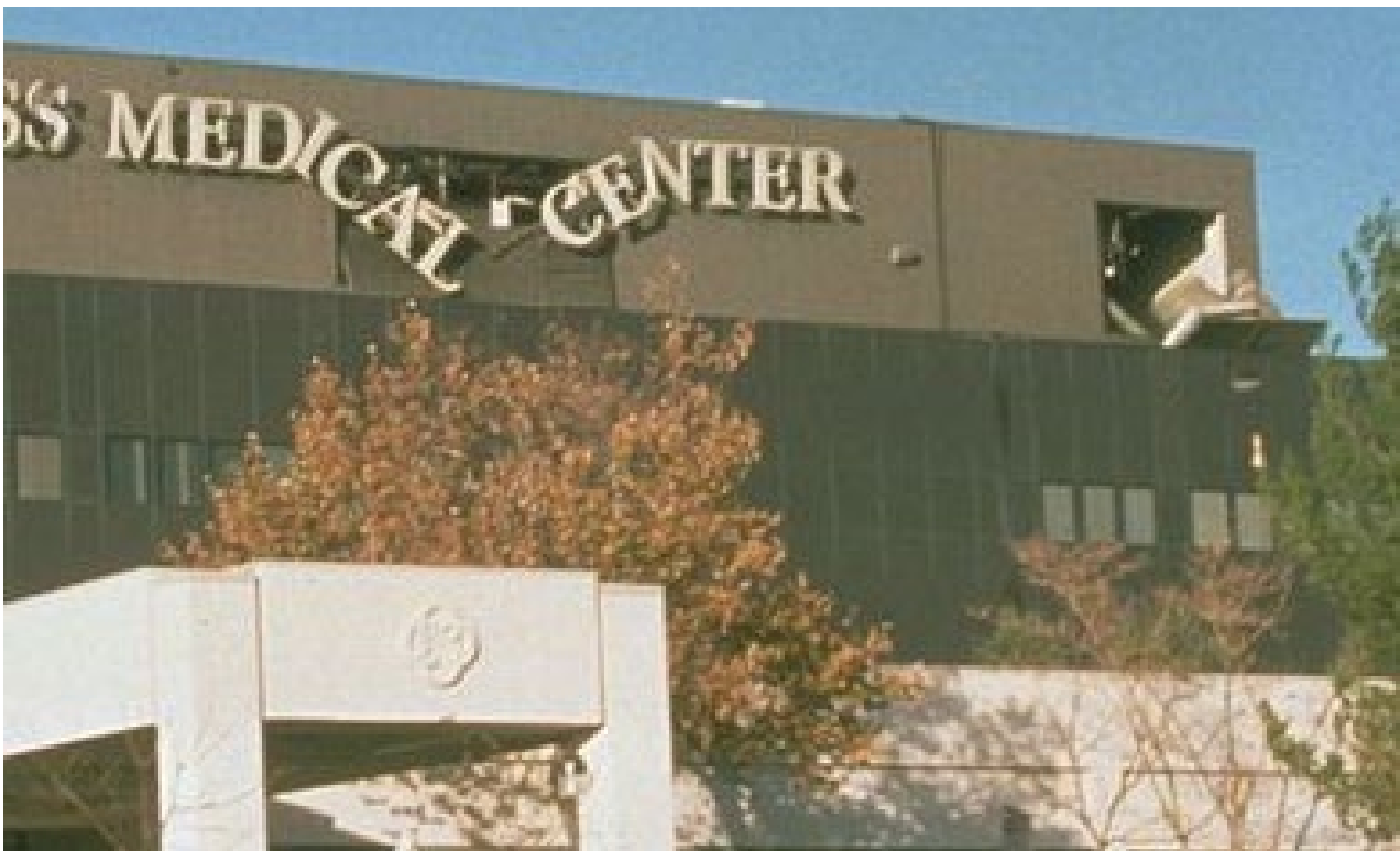
Figure 4-3. The 1994 Northridge Earthquake seemingly only cosmetically damaged this hospital's sign, but the cause was lunging of inadequately restrained air conditioning equipment that disabled the functioning of the facility. (Source: Robert Reitherman)
