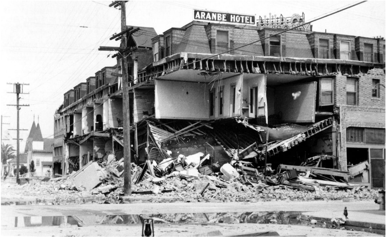
Figure B-1. The March 10, 1933 Long Beach Earthquake in Southern California was the impetus for development and adoption of building code regulations in the United States. (Source: Los Angeles County Library )
