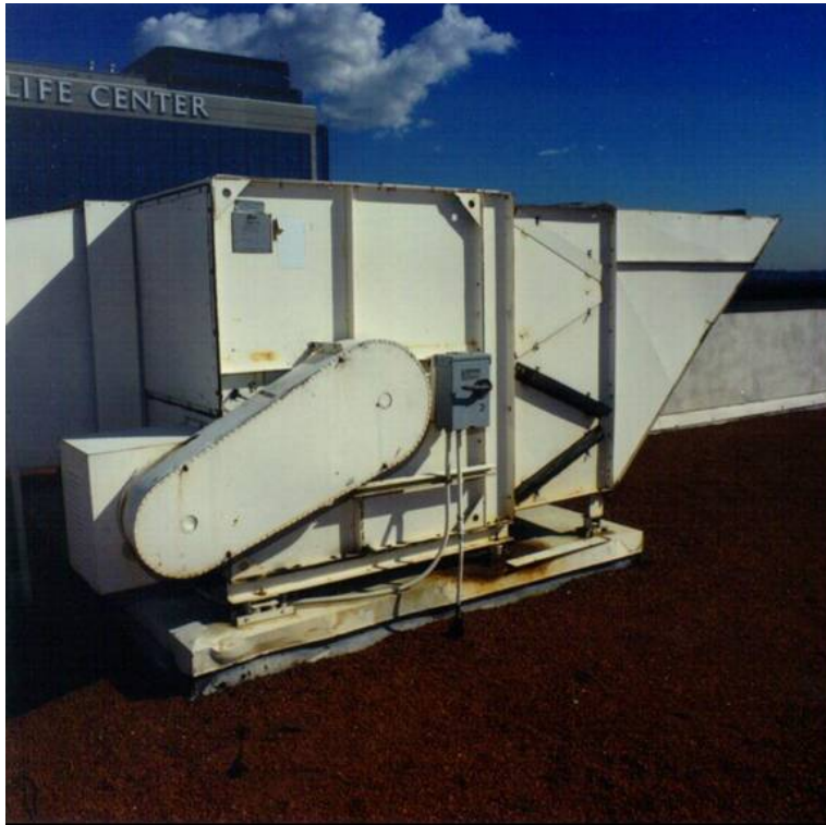
Figure 6.1-3 Fan Enclosure
