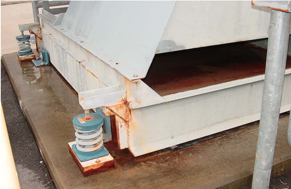
Figure 6.2-8 Side Bumpers (Snubbers)
