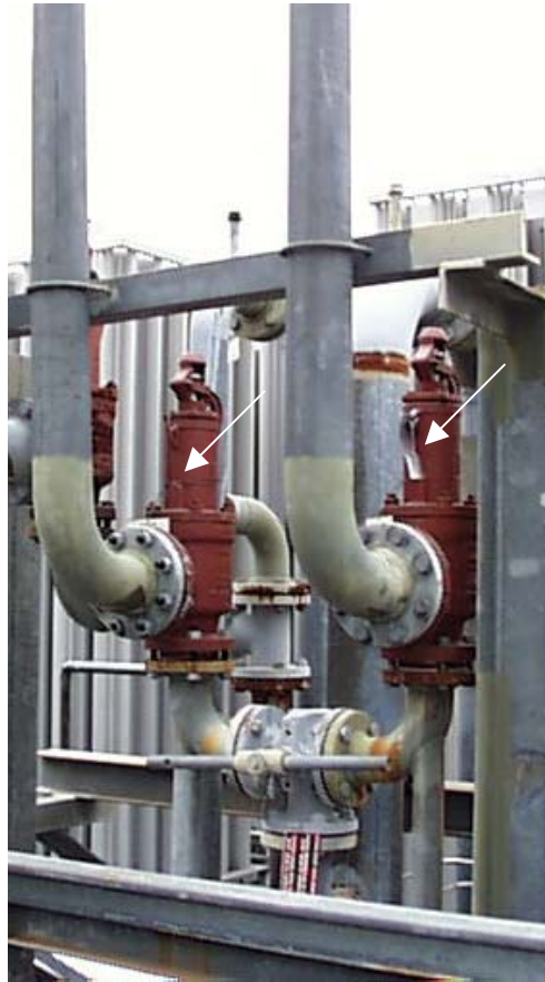
Figure 3.1-18 Pressure Relief Valves
