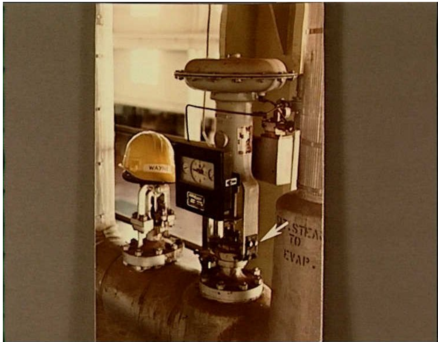
Figure 3.2-2 Repaired Cast Iron Yoke (ABS Consulting)
