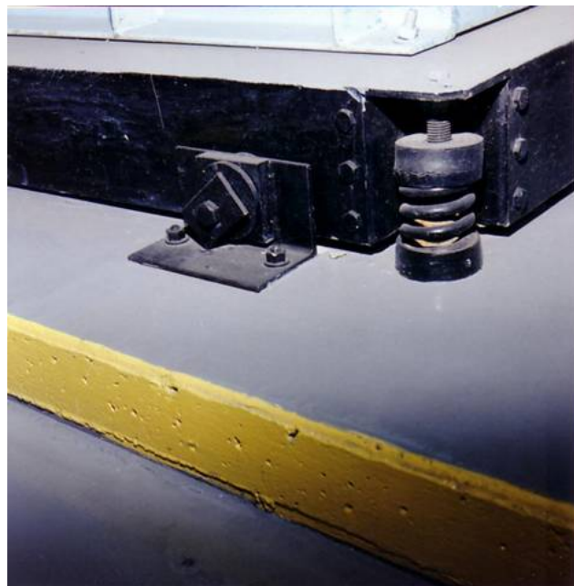
Figure 8.3-8 Seismic Snubber Separate from Isolators
