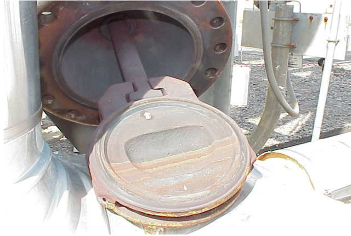
Figure 3.1-3 Valve Gate, Stem and Bonnet
