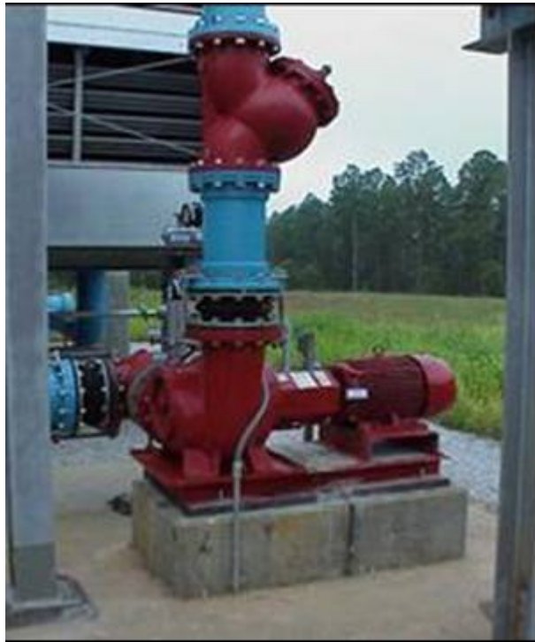
Figure 2.2-3 In-Line Check Valve
