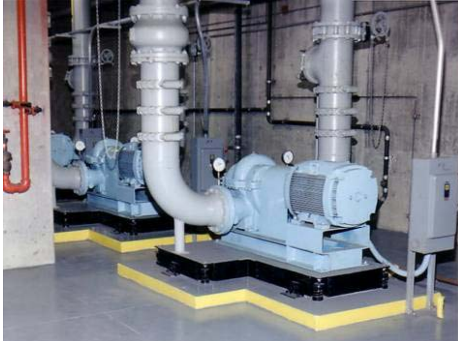
Figure 4.1-16 Centrifugal Pump and Motor on Common Pedestal (Mason Industries)
