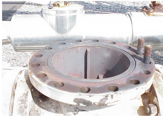
Figure 3.1-4 Valve Body and Gate Guide
