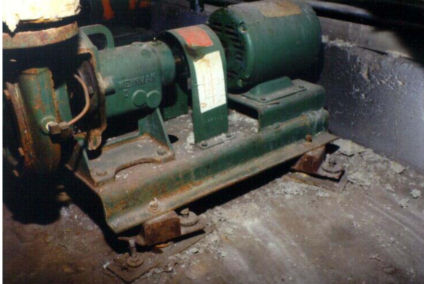
Figure 4.2-8 Pump Base Slides (Mason Industries)
