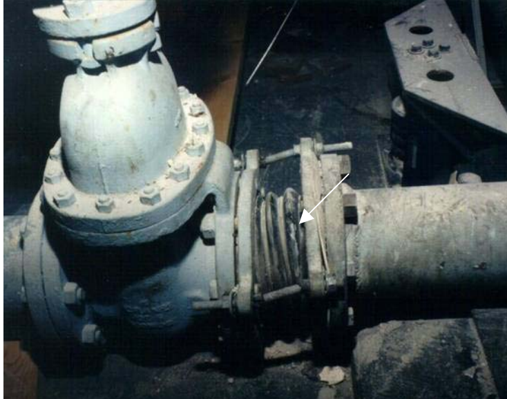
Figure 3.2-3 Bellows Joint at Valve-Pipe Nozzle (Mason Industries)
