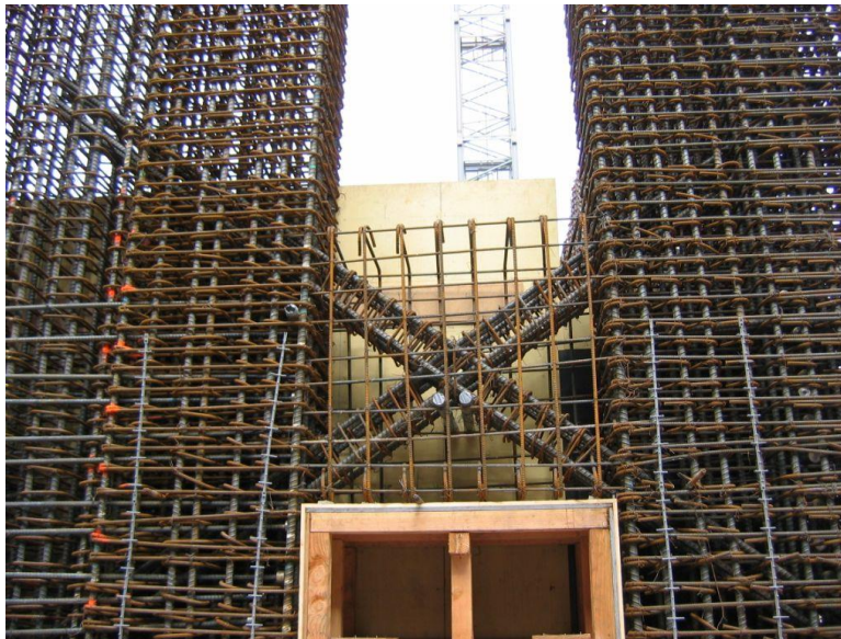
Figure 2.1-8 A diagonally reinforced coupling beam (Source: http://nees.seas.ucla.edu/pankow )
